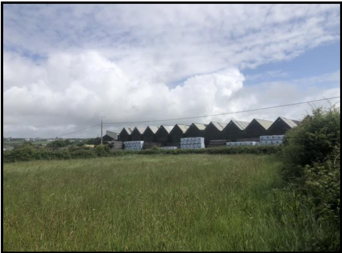
Plate 3.4 Looking east from the centre of the site
